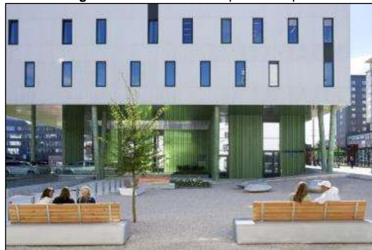
Figura 14 – Fachada Principal do Hospital
