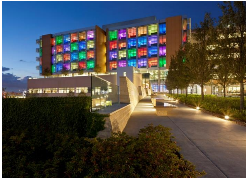
Figura 32: Fachada Principal do hospital
